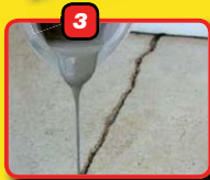
3 Pour mixture in the crack and level off with scraper
