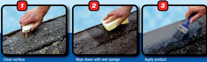
Use bridging fleece for cracks larger than 2mm (included in kit)
